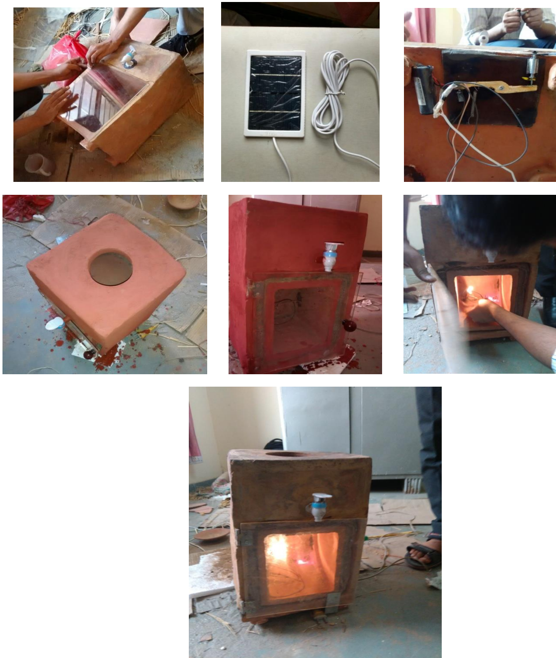
Fig.1. Process of construction “MITTI FRIDGE” installed with solar light.
