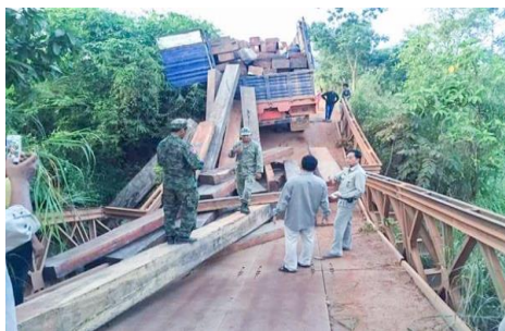
Bridge Broken by Illegal Load
